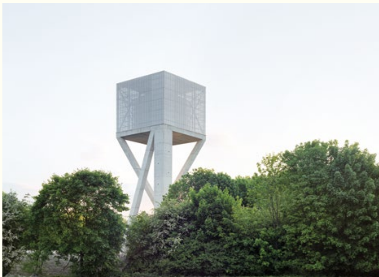
Construction of a 2,000 cubic metre water tower, Ghlin, Hainaut, 2014. The 20-metre-diameter circular tank is displayed on a 50-metre-high table. The four concrete legs cast on site are formed by the intersection of an X and a V.
